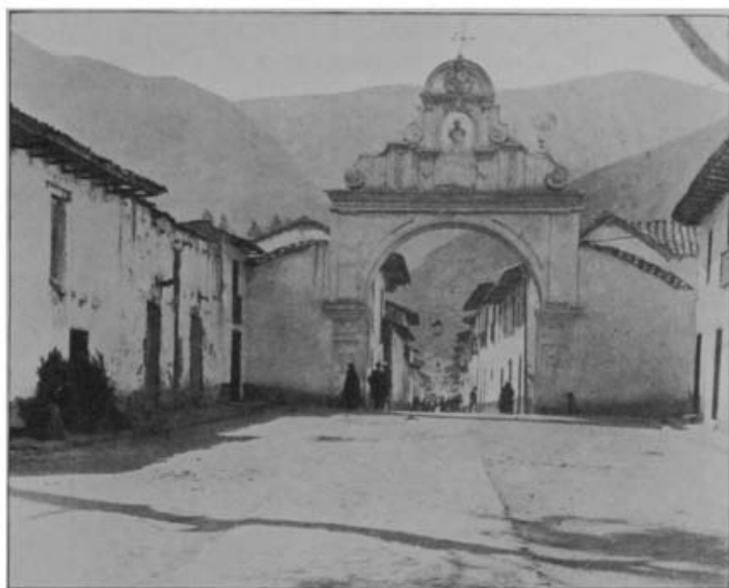
TARMA GATEWAY ON THE OROYA ROAD
