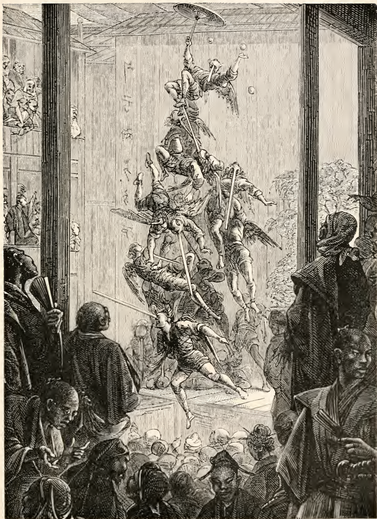
THE MONUMENT COLLAPSED LIKE A CASTLE OF CARDS.
