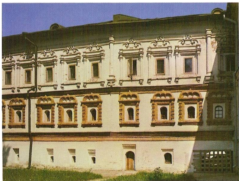
Корпус над погребами Ипатьевского монастыря. XVI—XVIII Building over the cellars in the Ipatievsky Monastery. 16th — 18th centuries
