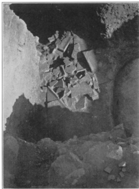
FIGURE 38. VIEW OF A SECTION OF THE LAYER OF ROOF TILES. TAKEN FROM ABOVE
