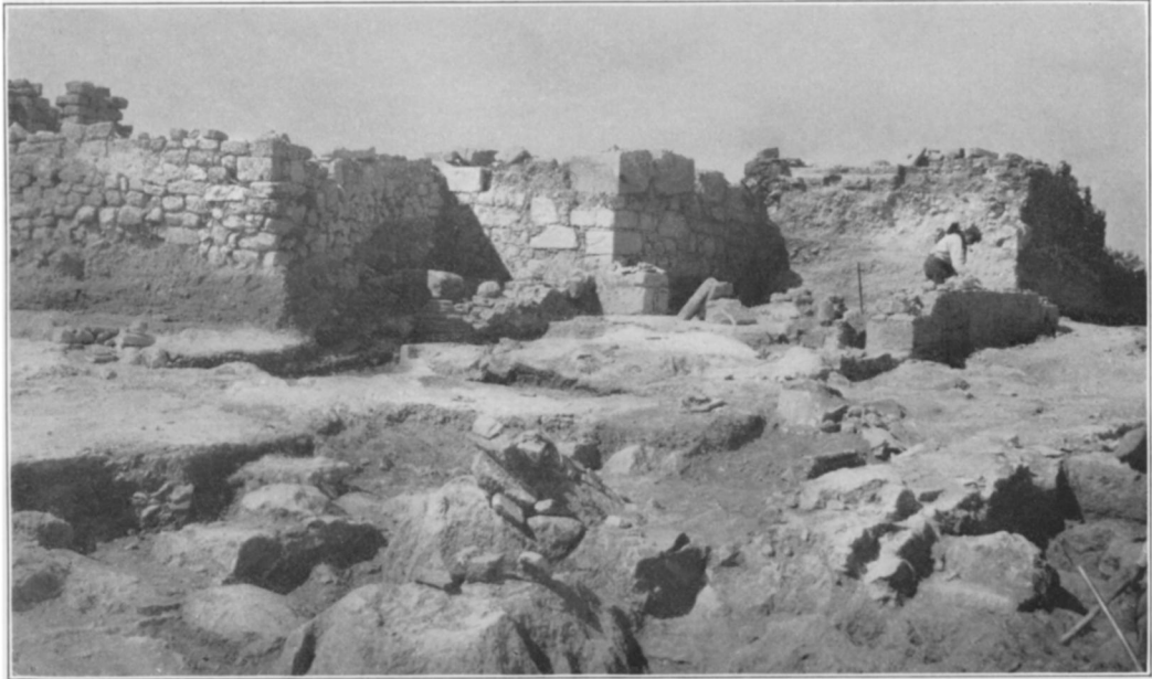
FIGURE 1. GENERAL VIEW ACROSS NAVE OF CHURCH, SHOWING ACCUMULATION OF EARTH AGAINST NORTH SIDE OF TOWER
