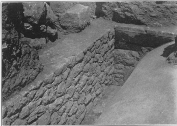
FIGURE 42. WEST RETAINING WALL
