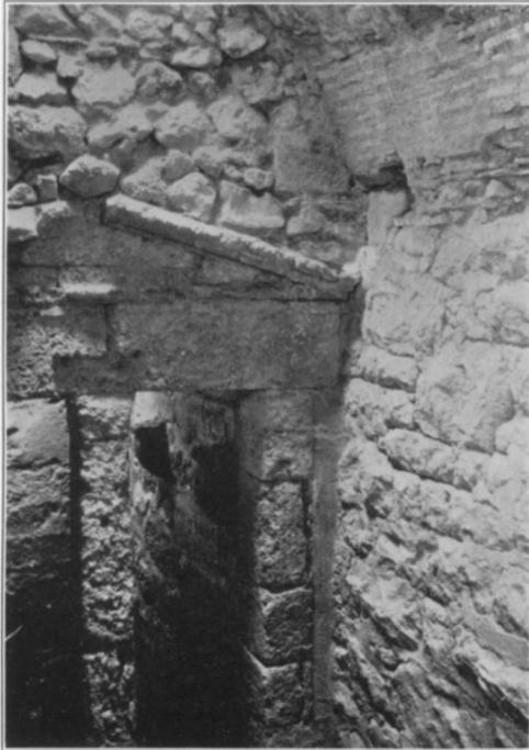
FIGURE 45. SCREEN SEEN FROM OUTER CHAMBER, SHOWING THE UPPER PART OF CHAMBER WALL AND THE REMAINING COURSES OF THE ROMAN BRICK VAULT
