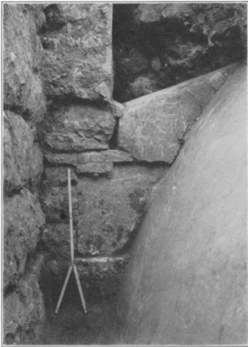
FIGURE 48. END OF ARCHITRAVE BACKERS SEEN FROM OUTSIDE OF VAULT
