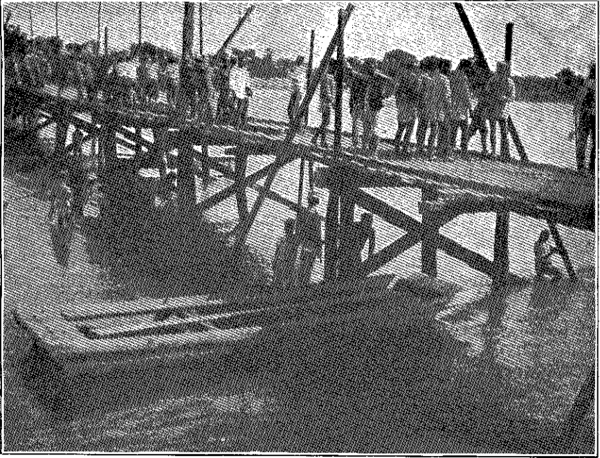
15. BUILDING BRIDGE ACROSS HAICHENG RIVER.
