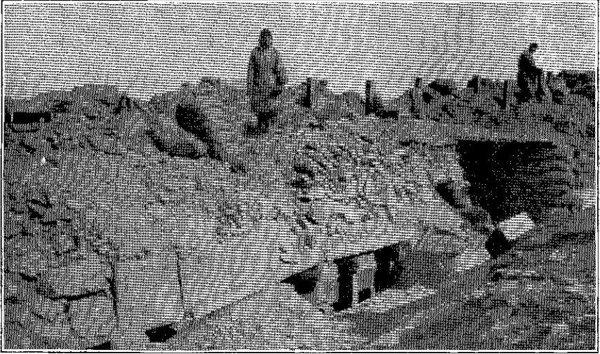
61. CHINESE WALL AT "H," SHOWING RUSSIAN BOMBPROOFS UNDER PARAPET.
