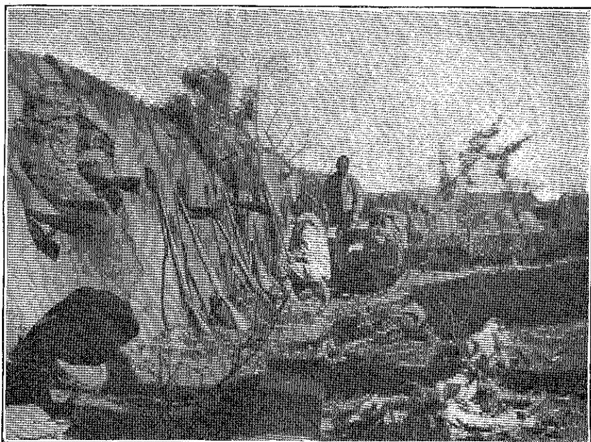
39. PREPARED WALL, LINSHENGPU, SHA RIVER.
