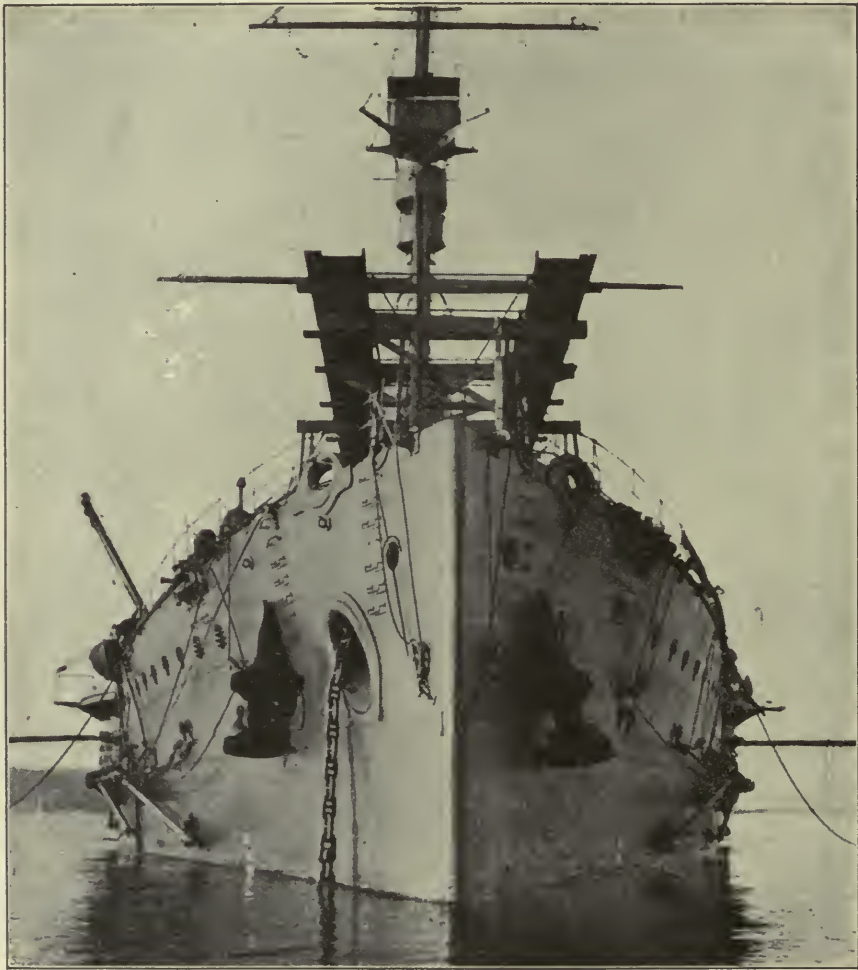
Bow of a British Dreadnought with Launching Platform for Aëroplanes
