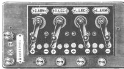
Fig. 108.—Special Commutator for a 4-Cell Schnee Bath.
