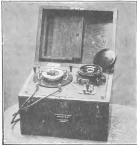
Fig. 92.—Galvanic Battery with Collector and Commutator.
