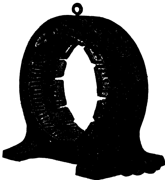
FIG. 14—DETAIL VIEW OF THREE-PHASE CONCENTRIC WINDING
