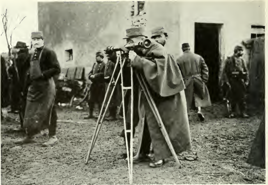
Range finding with the telemeter as used in the French army.
