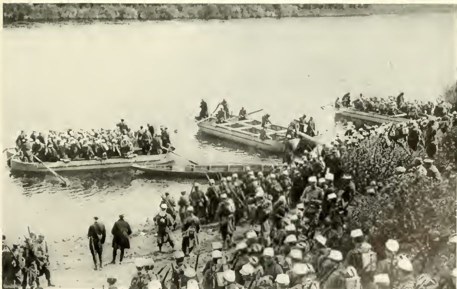
French Army : pontoons used for ferrying troops across a river or for constructing a floating bridge.
