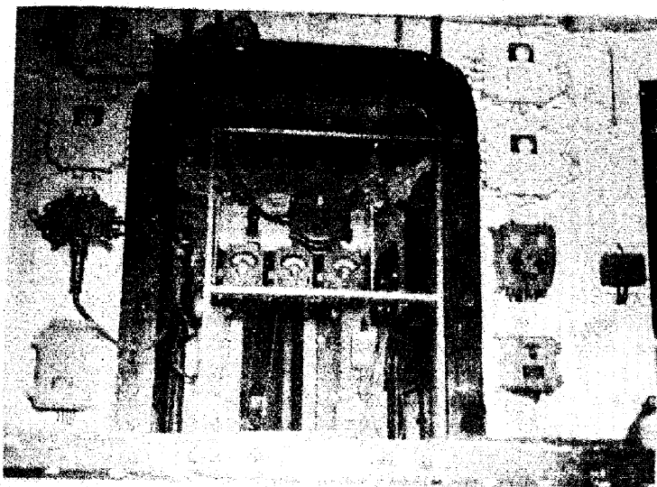
Fig. 18. Turret Control station, for all turret guns Note the duplicate azimuth and range potentiometer meters and the signaling telegraph
