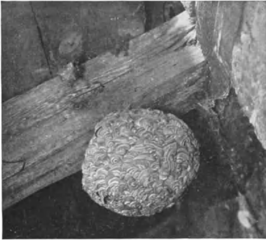
Abb. 75. Wespennest an einem Balken (nach Bischoff).
