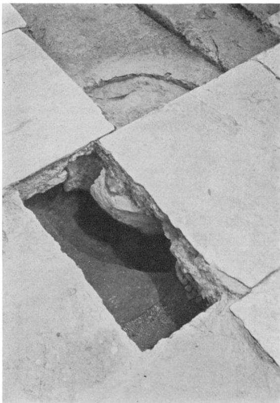
Fig. 69. Drain Channel in East Central Column of Tholos, from Southwest
