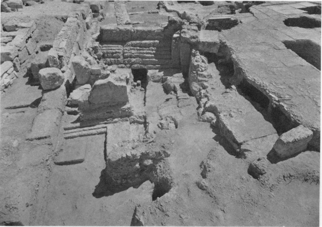
Fig. 57. Area of Tholos Kitchen from West
