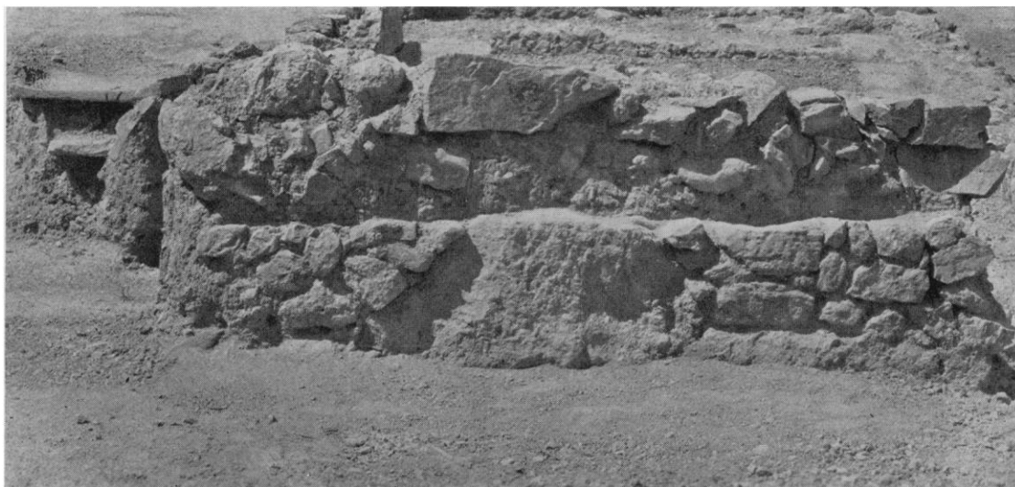
Fig. 15. East Wall of Building F, with Early Enclosure Wall Above and Drain of Tholos Kitchen to Left, from East
