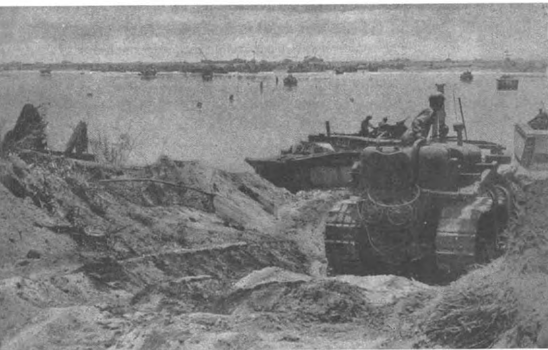
BULLDOZERS CLEARED ROADS to beach dumps for the tracked amphibious vehicles which carried the supplies from the reef to storage and dispersal areas on shore. Along the reef (at center) a crane loads a tractor; the transport ships are anchored farther out to sea.
