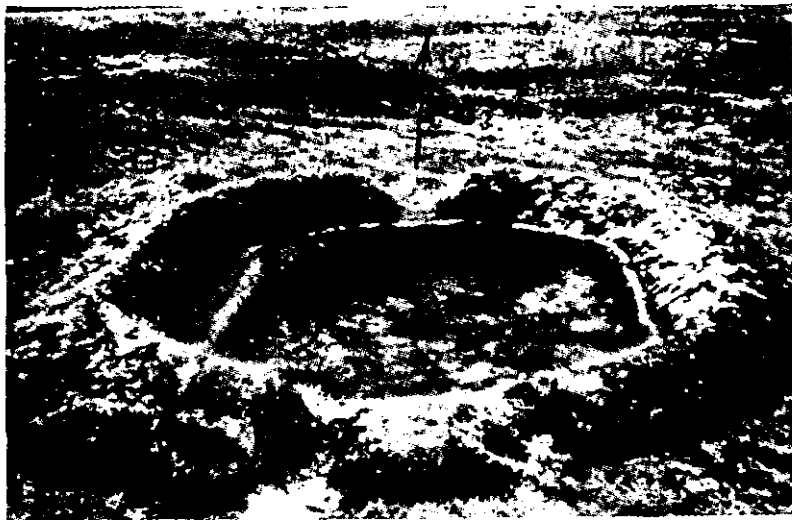
Figure 46.—Emplacement for antitank gun in flat terrain.
