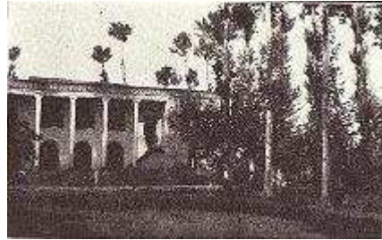
Some of the American Mission buildings destroyed by the Moslems. Courtesy, Near East Relief.
