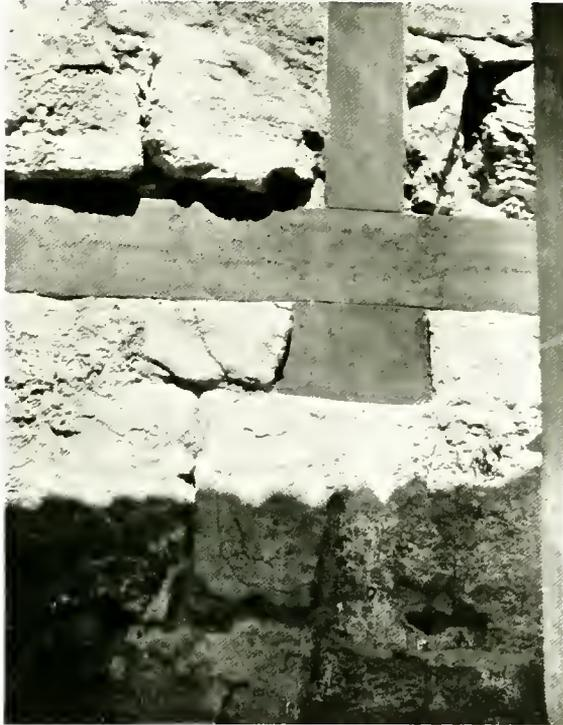
*a.* VERTICAL POST (SOCKETED IN M. M. II MASONRY) WITH BASE TAPERING UPWARDS. EAST CORRIDOR. (See p. 65.)
