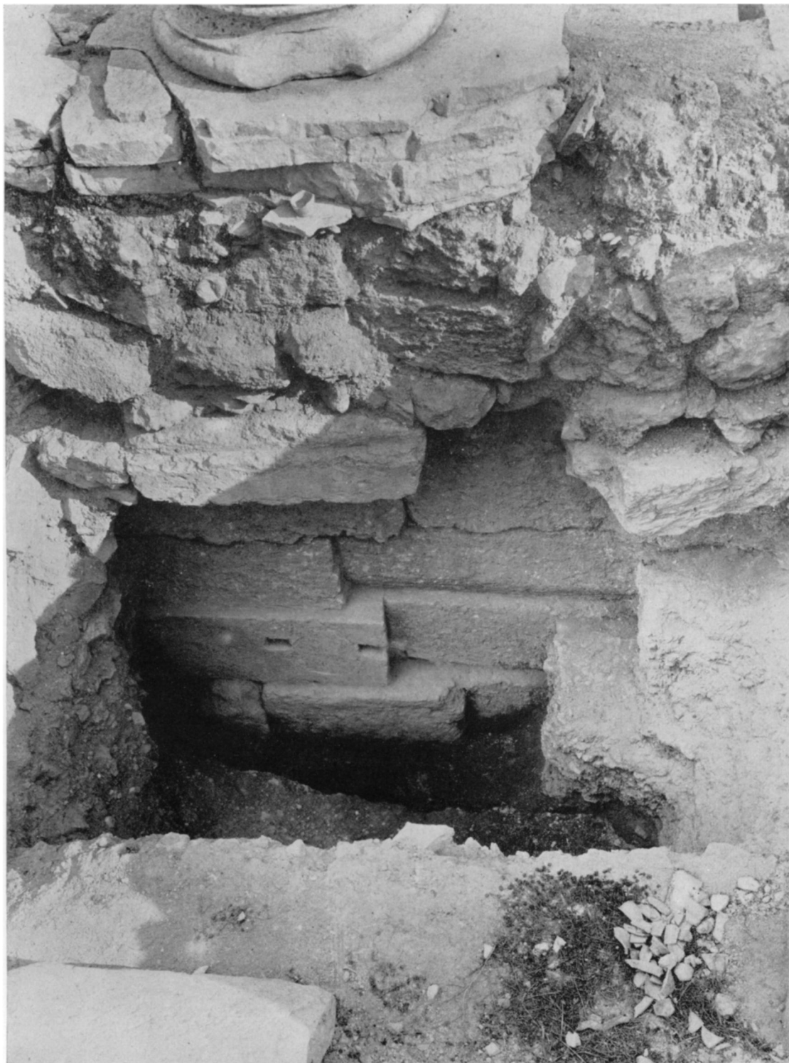
Fig. 13. Foundation of Stylobate of Hellenistic Stoa. At the Top Is the Stylobate of the Marble Peribolos with Its Rubble Concrete Foundations
