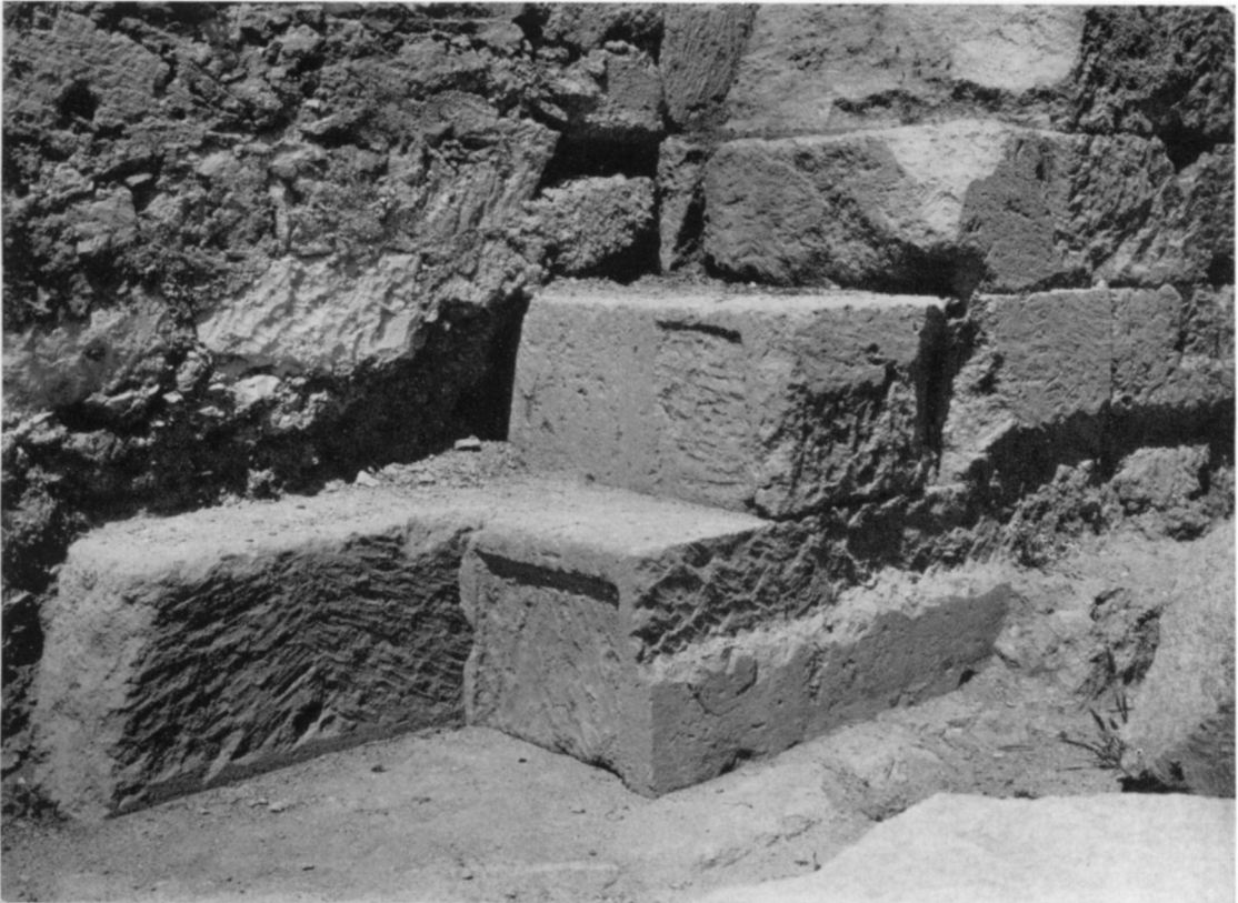
Fig. 119. Blocks Near the East End of the South Side of the Podium, Showing Cutting for Base Moulding
