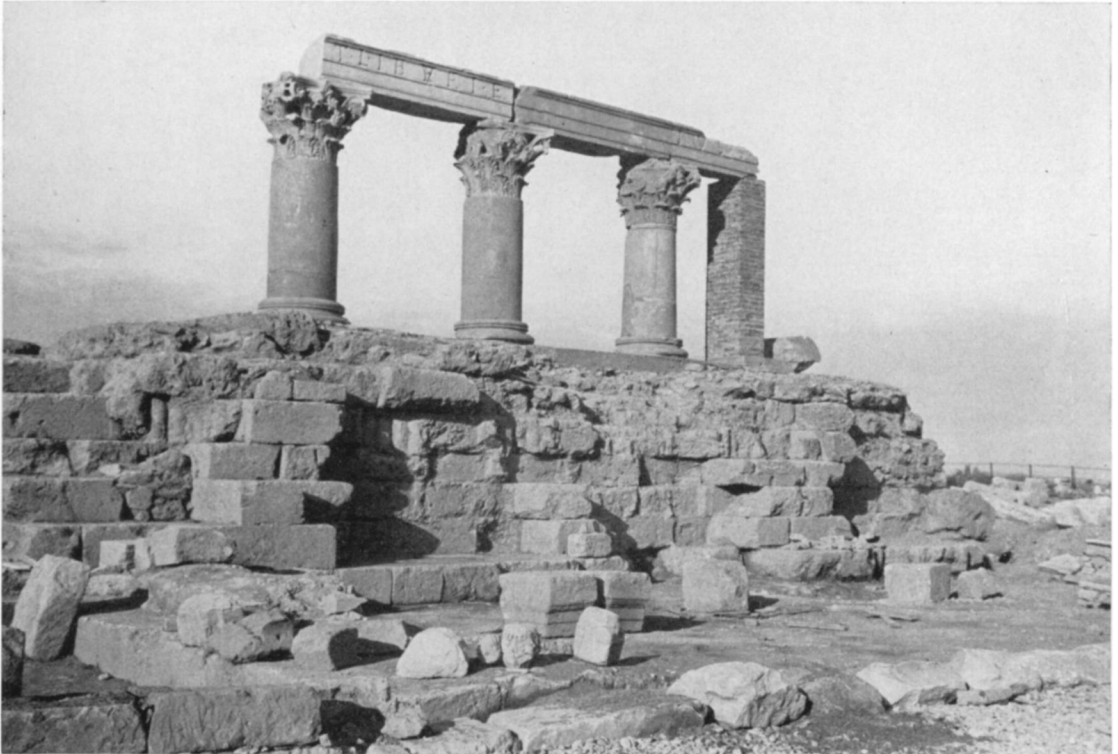
Fig. 107. East End of the Podium
