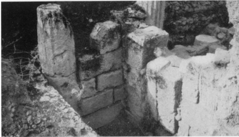
Fig. 84. Construction at Juncture of Narrow West Chamber of Shops and Colonnade of Stoa. The Door, Cut to Gain Access to the Latrine, Was Later Blocked
