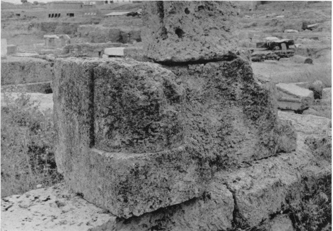
Fig. 96. The Applied Column Drum in Situ on the Front Wall of the Precinct
