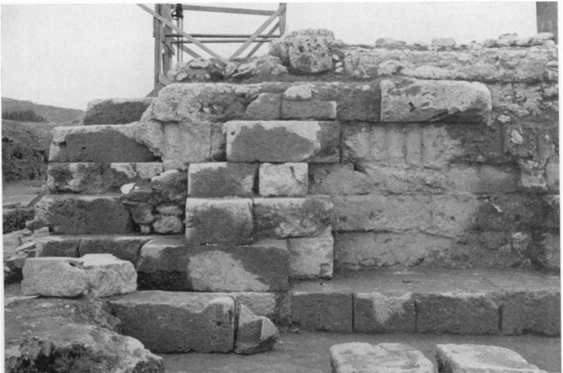
Fig. 117. Southeast Corner of the Podium
