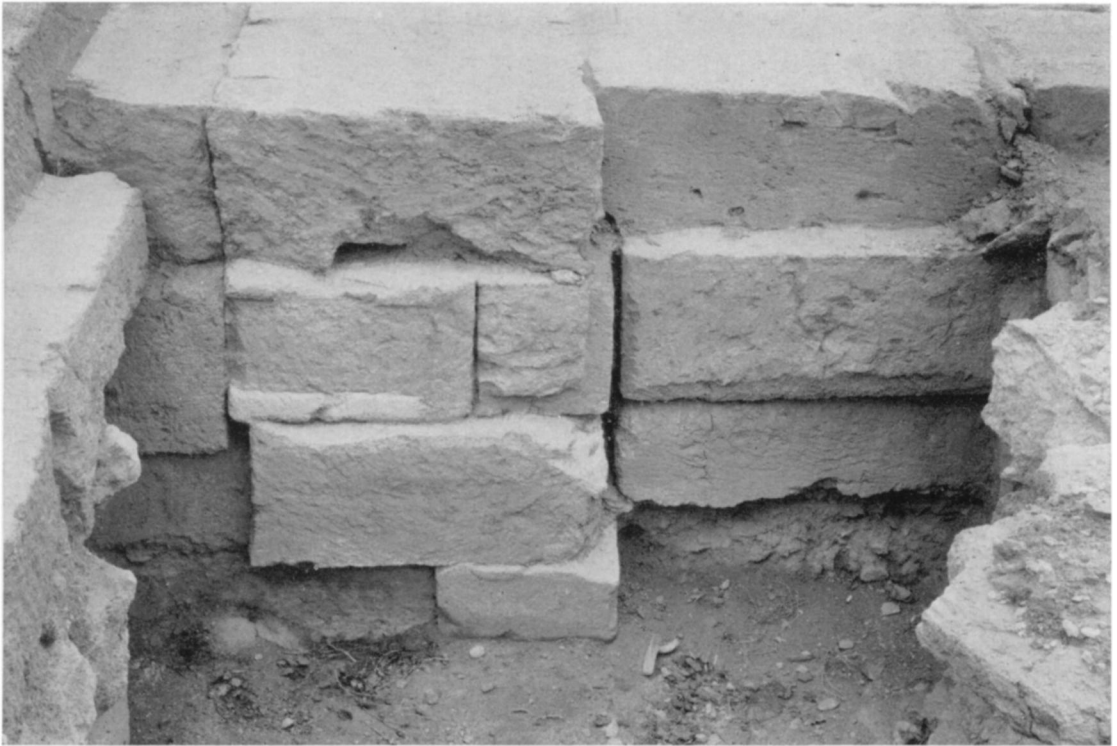
Fig. 116. Foundation Under Southwest Corner of Podium
