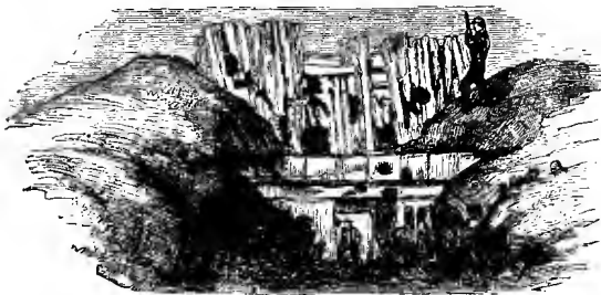
CASEMATE NO. 1 DESTROYED BY THE U. S. GUN-BOAT "BARON DE KALB."
