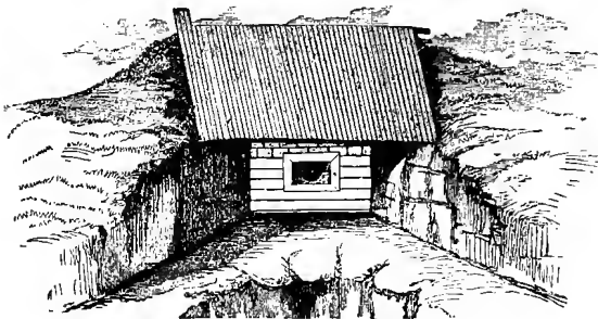
APPEARANCE OF CASEMATES BEFORE THE ATTACK (COVERED WITH RAILROAD IRON).
