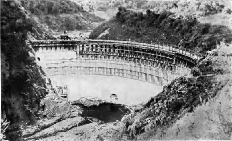
Abb. 148. Carmel River Dam.
