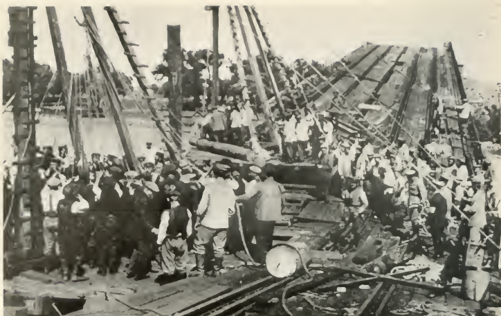
German pioneers repairing one of the bridges across the Vistula which had been blown up by the Russians on their retreat.
