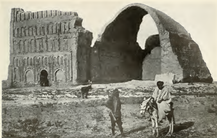
The great arch at Ctesiphon. Remains of the palace of Takhti Khesra, built by Chosroes I, A. D. 550 The arch, built of brick, is eighty-three feet wide and ninety-five feet high.
