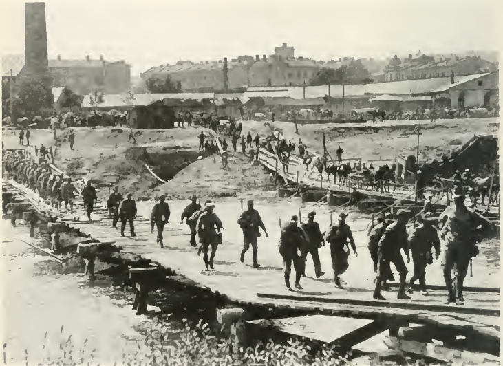
Austrian troops crossing the River San. As the Russians retreated they of course destroyed the bridges. Above is shown two types of military bridges, one of pontoons on the right background, and one of driven piles in the foreground.
