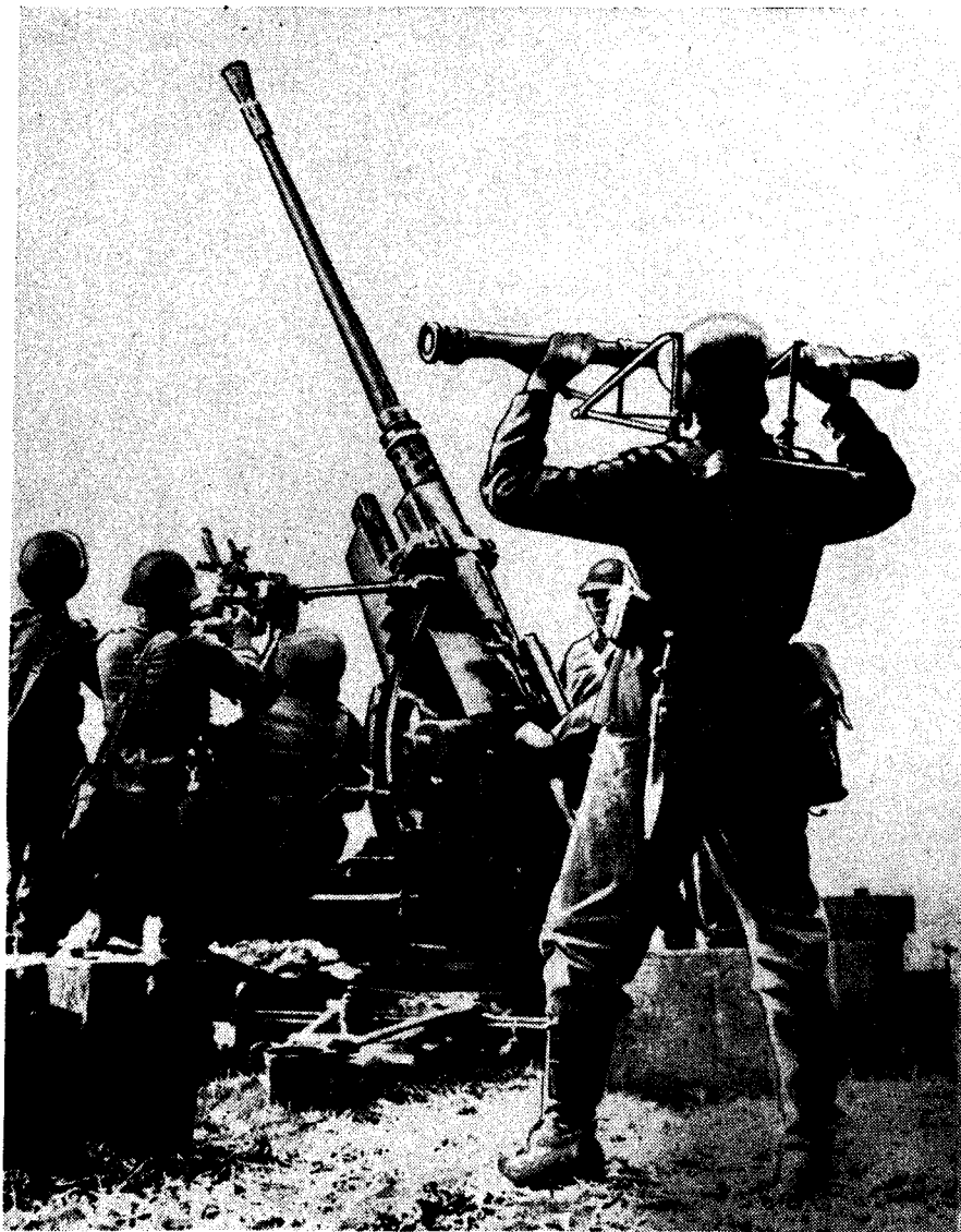
Figure 7.—1-meter-base range-finder in use with 3.7-cm (37-mm) AA/AT gun.
