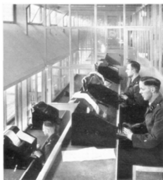
Telewriting machines at the Directing Headquarters in the Olympic Stadium.
