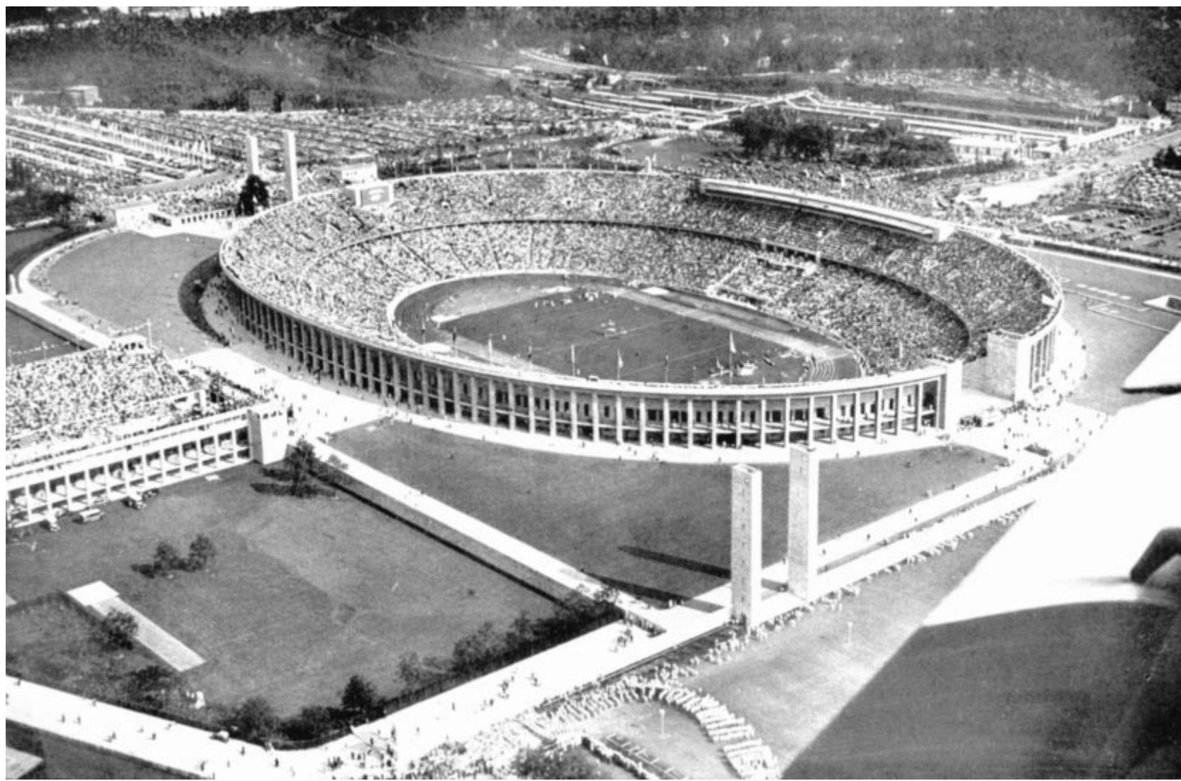
The Olympic structures, close to the edge of the city, and the streets leading to the Olympic Stadium.
