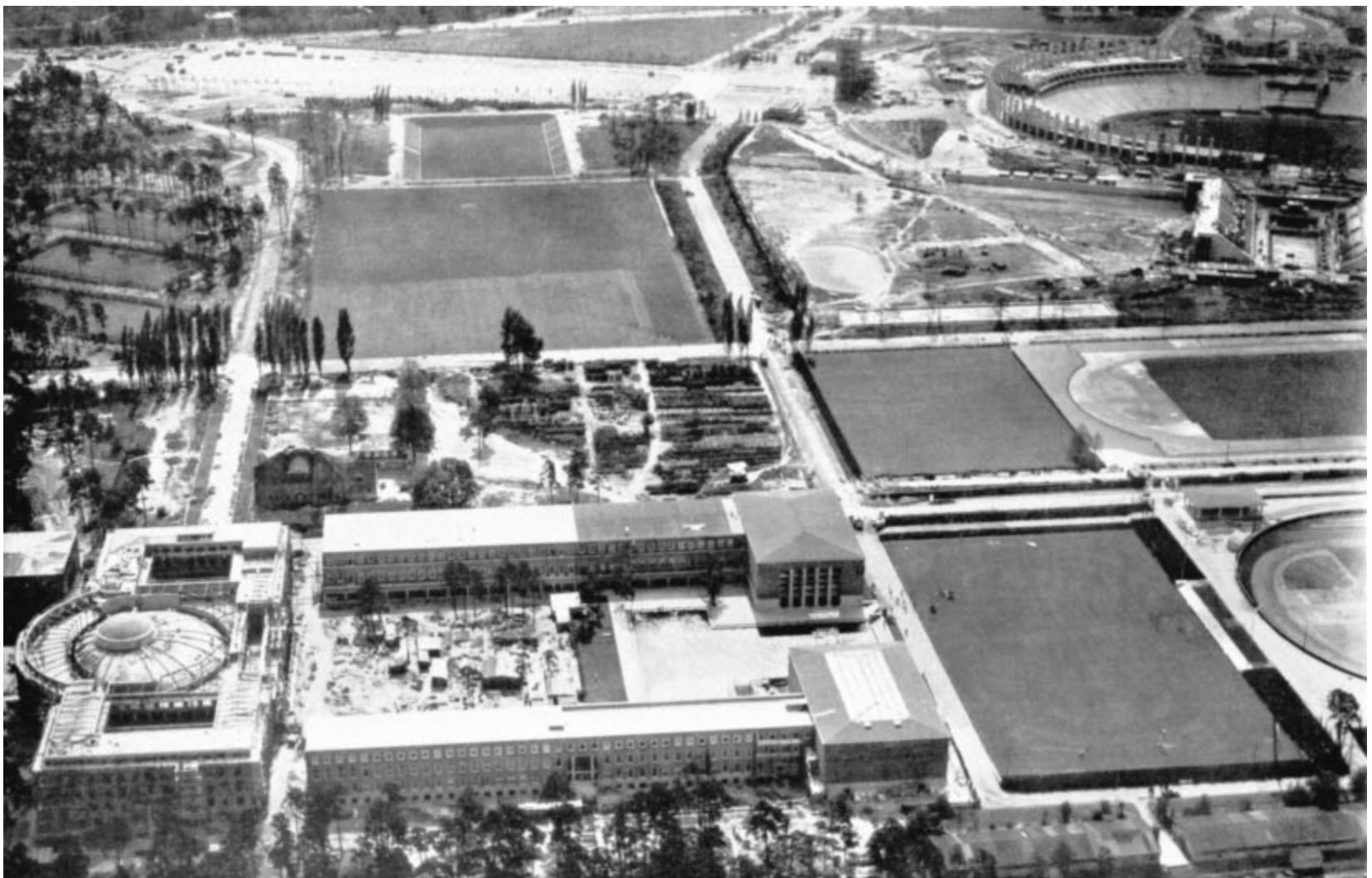
The Reich Sport Field during construction. Lower left: the Cupola Hall of the House of German Sport, the site of the Olympic fencing tournament. Upper right: the Olympic Stadium.
