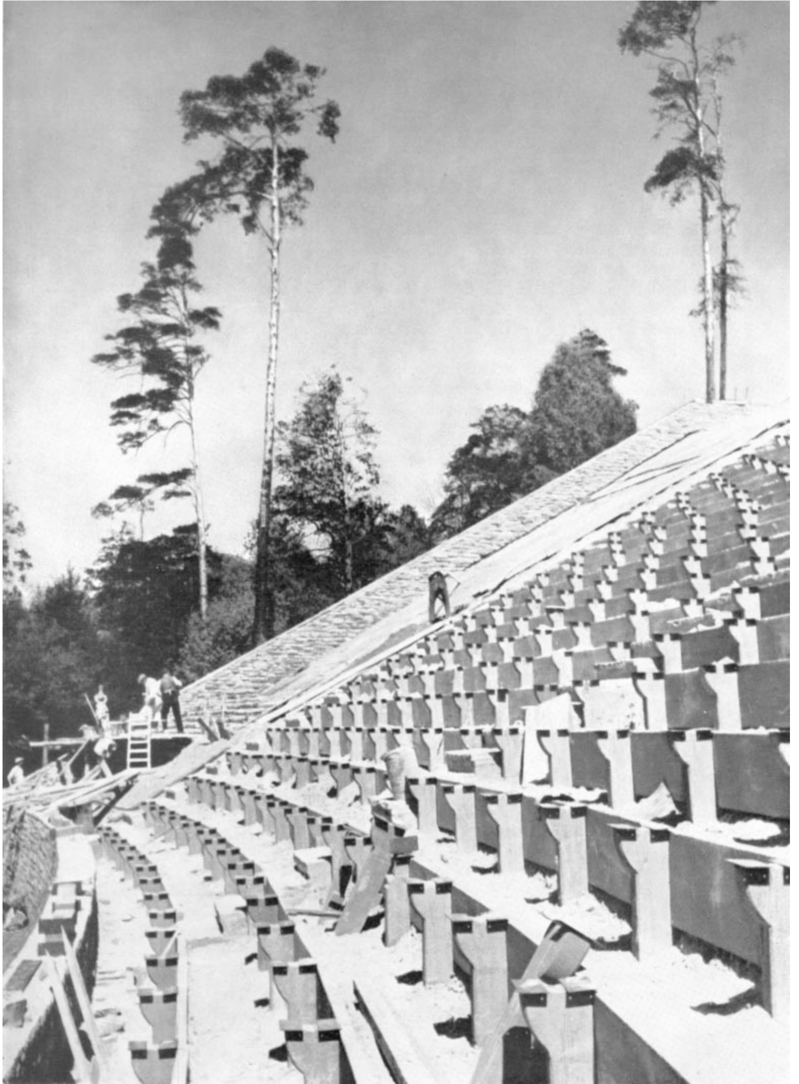
The Olympic amphitheatre, the Dietrich Eckart Open-Air Theatre, under construction.
