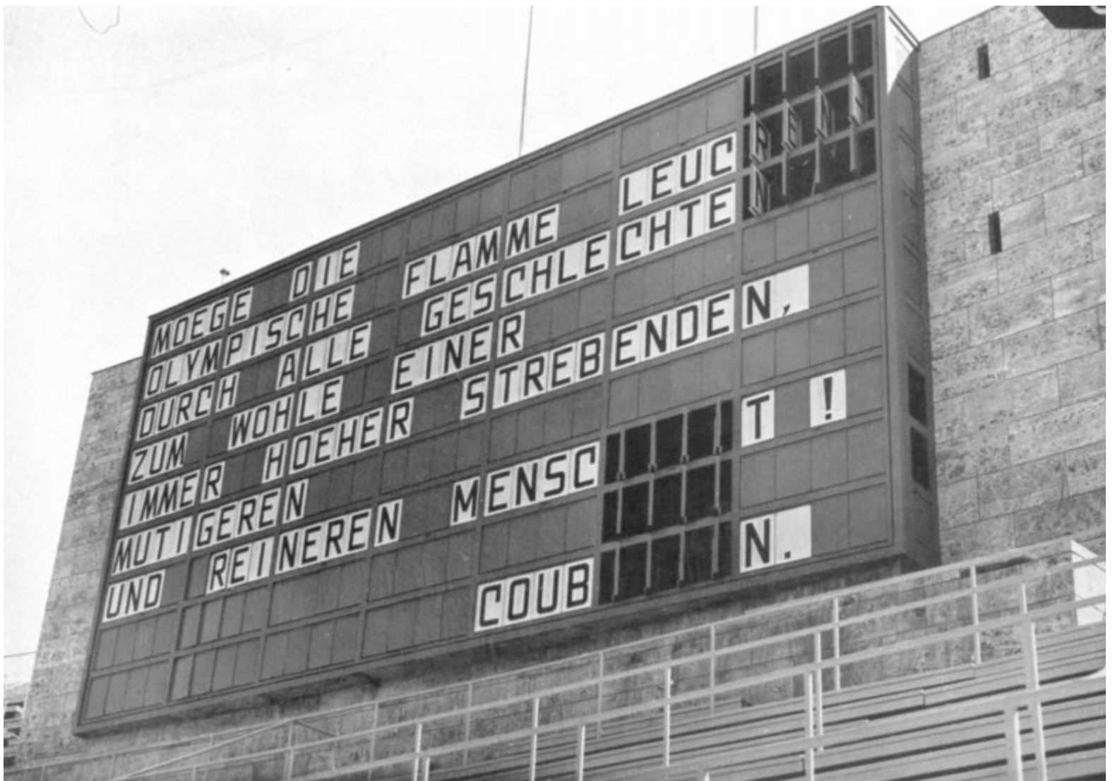
The announcement board at the eastern end showing the manner in which the letters are attached to revolving plates.
