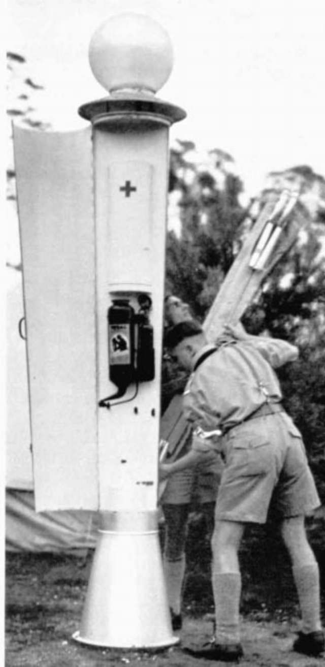
A "first aid beacon" at the International Youth Encampment containing a stretcher, first aid material and a fire extinguisher.
