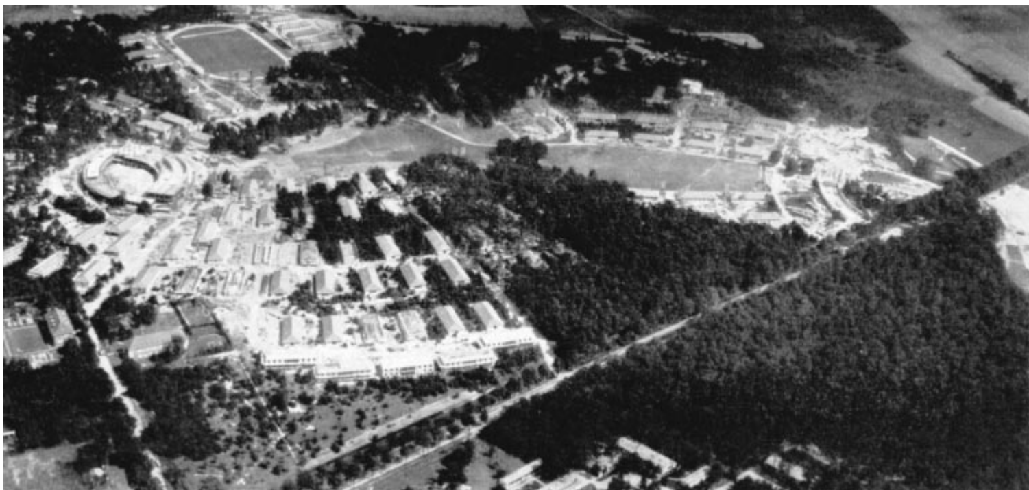
Bird's eye view of the Olympic Village during construction.
