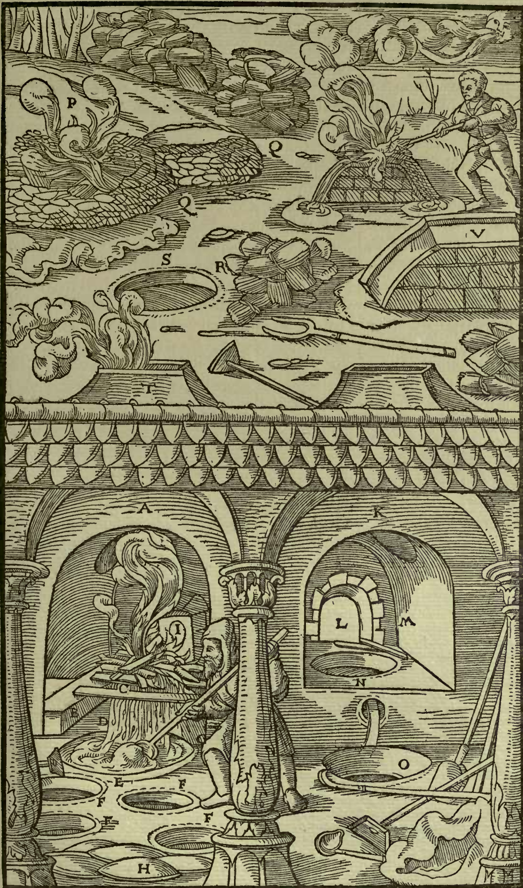
A—FURNACE OF THE CARNI. B—LOW WALL. C—WOOD. D—ORE DRIPPING LEAD. E—LARGE CRUCIBLE. F—MOULDS. G—LADLE. H—SLABS OF LEAD. I—RECTANGULAR HOLE AT THE BACK OF THE FURNACE. K—SAXON FURNACE. L—OPENING IN THE BACK OF THE FURNACE. M—WOOD. N—UPPER CRUCIBLE. O—DIPPING-POT. P—WESTPHALIAN METHOD OF MELTING. Q—HEAPS OF CHARCOAL. R—STRAW. S—WIDE SLABS. T—CRUCIBLES. V—POLISH HEARTH.
