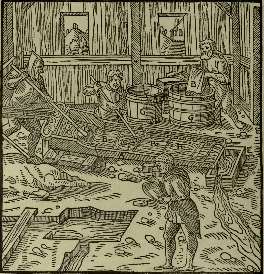
A—BEAMS. B—CANVAS. C—HEAD OF STRAKE. D—SMALL LAUNDER. E—SETTLING PIT OR TANK. F—WOODEN SCRUBBER. G—TUBS.
