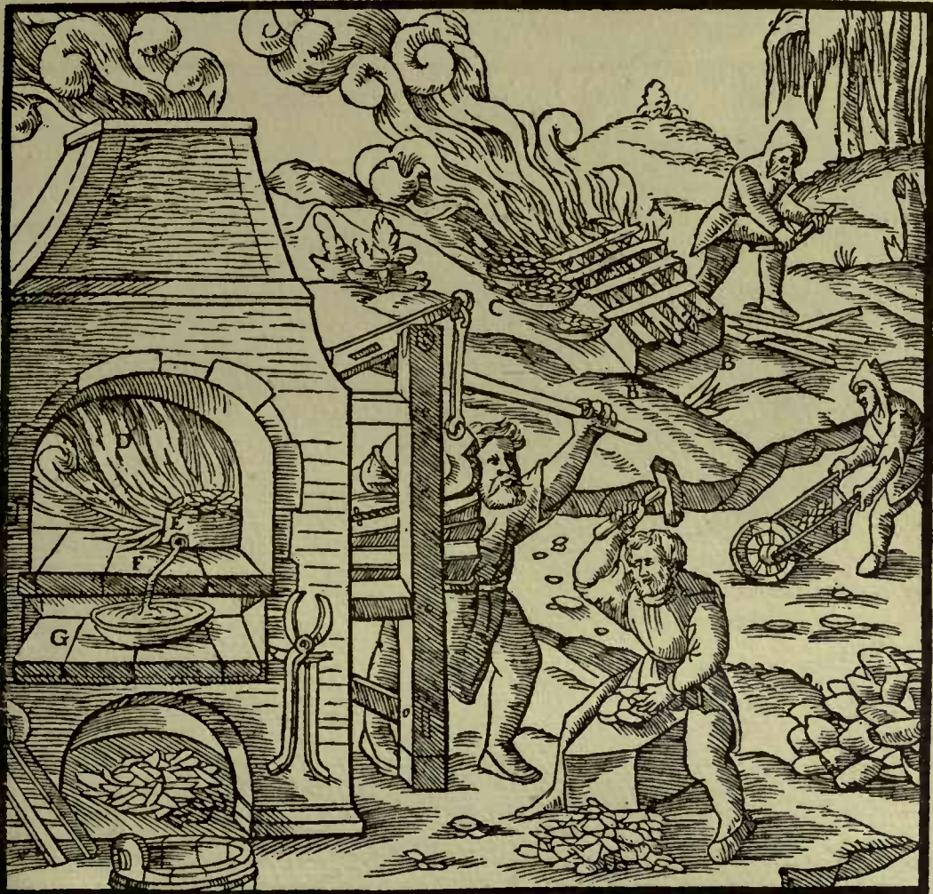
A—WOOD. B—BRICKS. C—PANS. D—FURNACE. E—CRUCIBLE. F—PIPE. G—DIPPING-POT.
