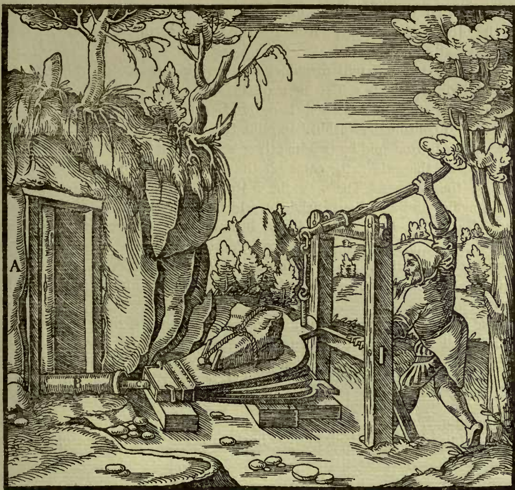
A—TUNNEL. B—PIPE. C—NOZZLE OF DOUBLE BELLOWS.
