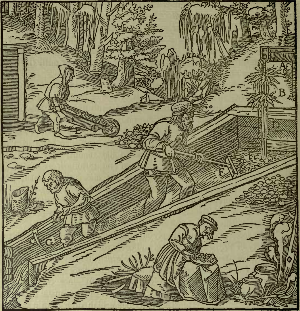
A—LAUNDER. B—INTERLACING FIR TWIGS. C—LOGS; THREE ON ONE SIDE, FOR THE FOURTH CANNOT BE SEEN BECAUSE THE DITCH IS SO FULL WITH MATERIAL NOW BEING WASHED. D—LOGS AT THE HEAD OF THE DITCH. E—BARROW. F—SEVEN-PRONGED FORK. G—HOE.
