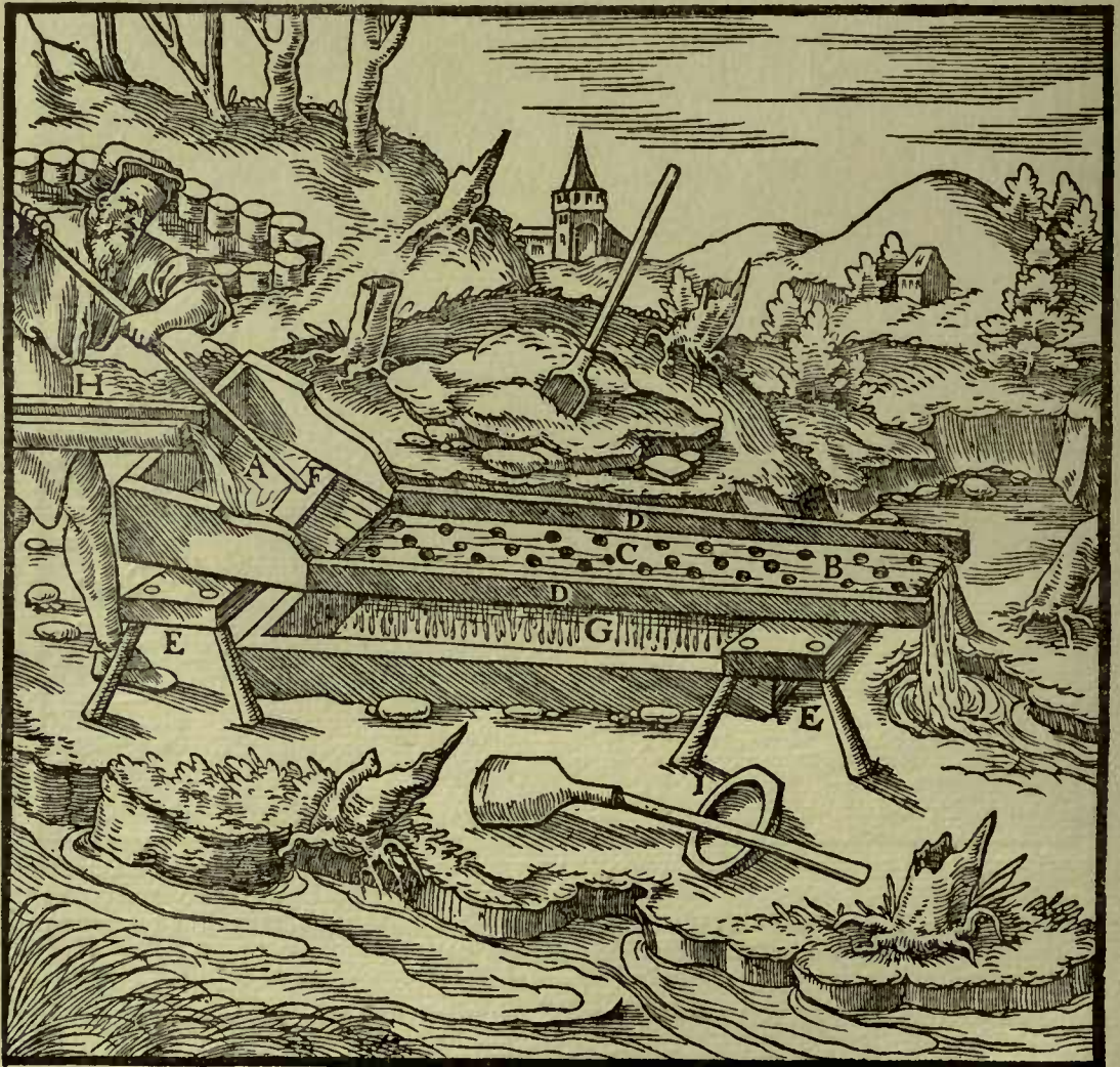
A—HEAD OF FRAME. B—FRAME. C—HOLES. D—EDGE-BOARDS. E—STOOLS F—SCRUBBER. G—TROUGH. H—LAUNDER. I—BOWL.
