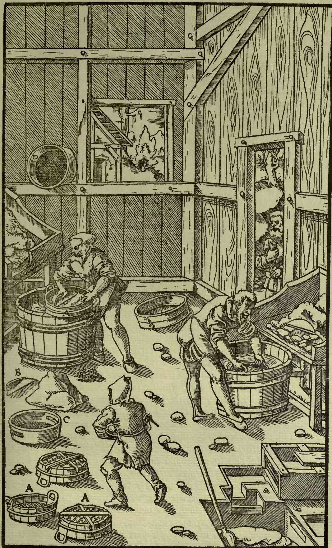
A—FINE SIEVES. B—LIMP. C—FINER SIEVE. D—FINEST SIEVE
