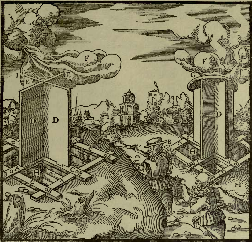
A—SILLS. B—POINTED STAKES. C—CROSS-BEAMS. D—UPRIGHT PLANKS. E—HOLLOW. F—WINDS. G—COVERING DISC. H—SHAFTS. I—MACHINE WITHOUT A COVERING.
