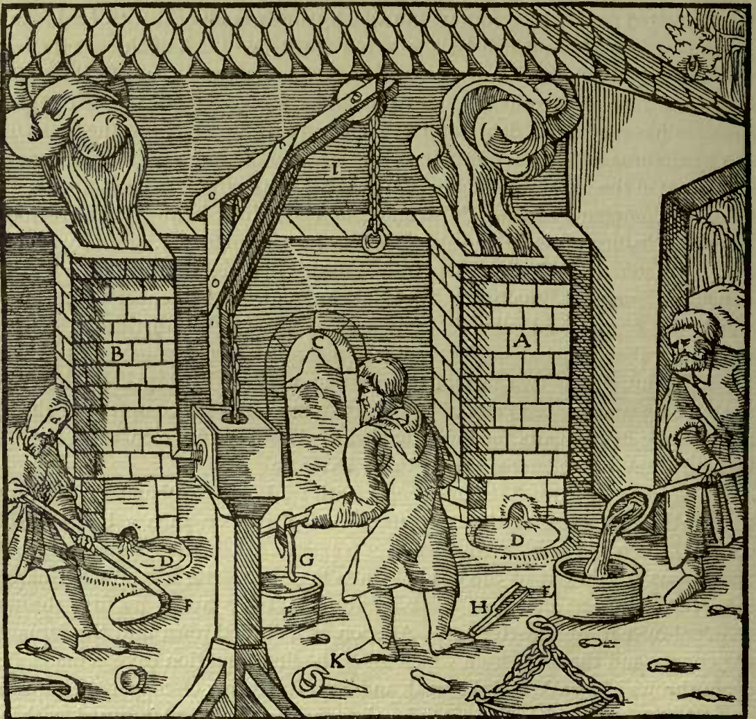
A—FURNACE IN WHICH "SLAGS" ARE RE-SMELTED. B—FURNACE IN WHICH COPPER IS ALLOYED WITH LEAD. C—DOOR. D—FORE-HEARTHS ON THE GROUND. E—COPPER MOULDS. F—RABBLE. G—HOOK. H—CLEFT STICK. I—ARM OF THE CRANE. K—THE HOOK OF ITS CHAIN.
