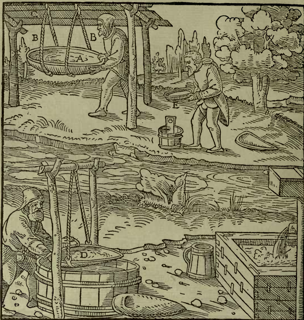
A—LARGE BOWL. B—ROPES. C—BEAM. D—OTHER LARGE BOWL WHICH COINERS USE. E—SMALL BOWL.
