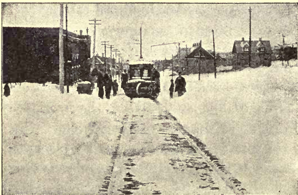
FIG. 140.—ELECTRIC SNOW SWEEPER.
