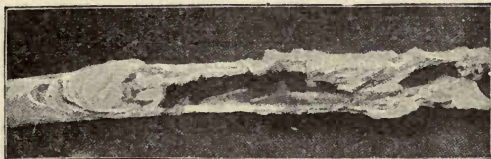
FIG. 124.—IRON PIPE CORRODED BY ELECTROLYSIS.
