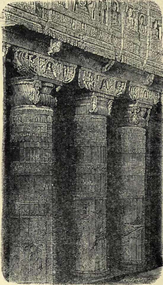
77. Pillars on the left side of the Nave, in Cave No. 26 at Ajantā. (From a Photograph.)
