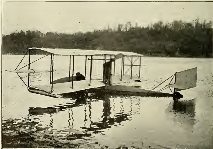
Detail view of the early Benoist Flying Boat. In later models the ailerons are fitted at the rear of the planes and a small fixed tail plane has been added. The motor, which is now a Sturtevant, is still carried in the hull, but the propeller position has been lowered somewhat.
