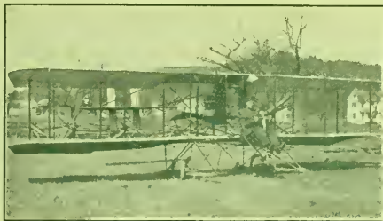
Earl V. Fritts' Thomas Biplane, equipped with 60-70 h. p. MAXIMOTOR
