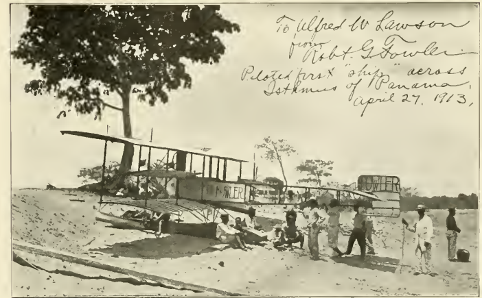
The above is a photograph of the hydro-aeroplane used by Robert G. Fowler in successfully crossing the Isthmus of Panama. Its power plant consisted of a 80 H. P. Hall-Scott motor.
