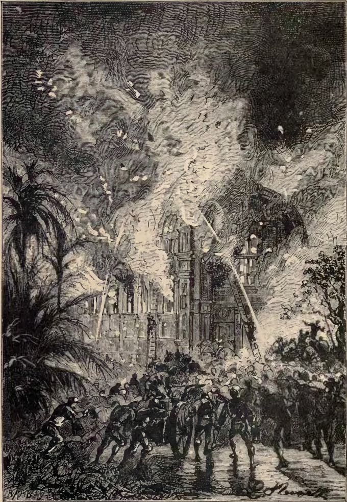
A destructive fire.
