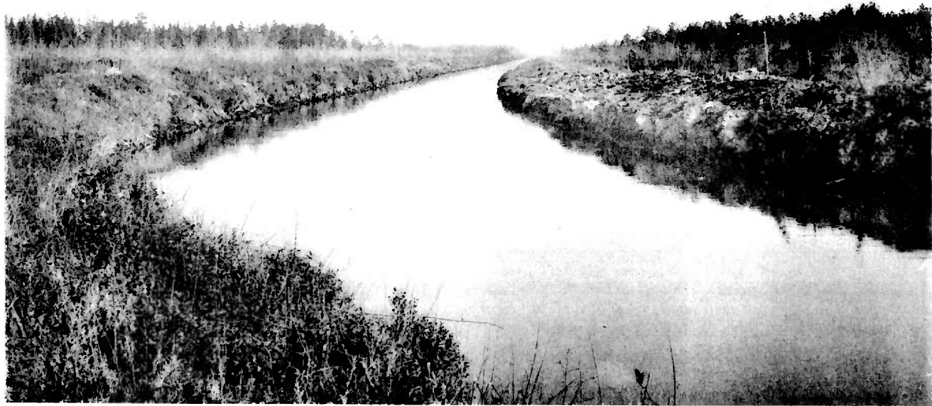
THE DISMAL SWAMP CANAL NEAR SOUTH MILLS, N. C.
