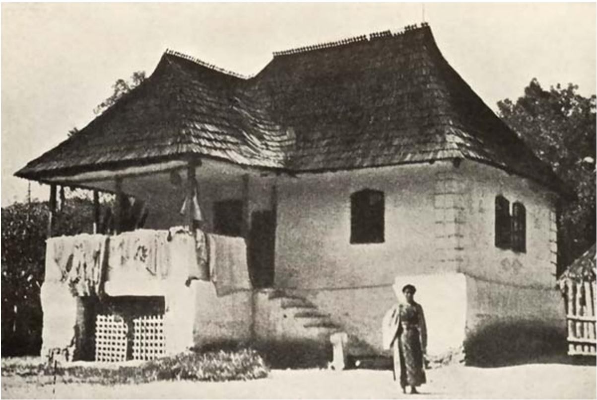
The thatched roofs are replaced by roofs of shingle that shine like silver in the sun.
