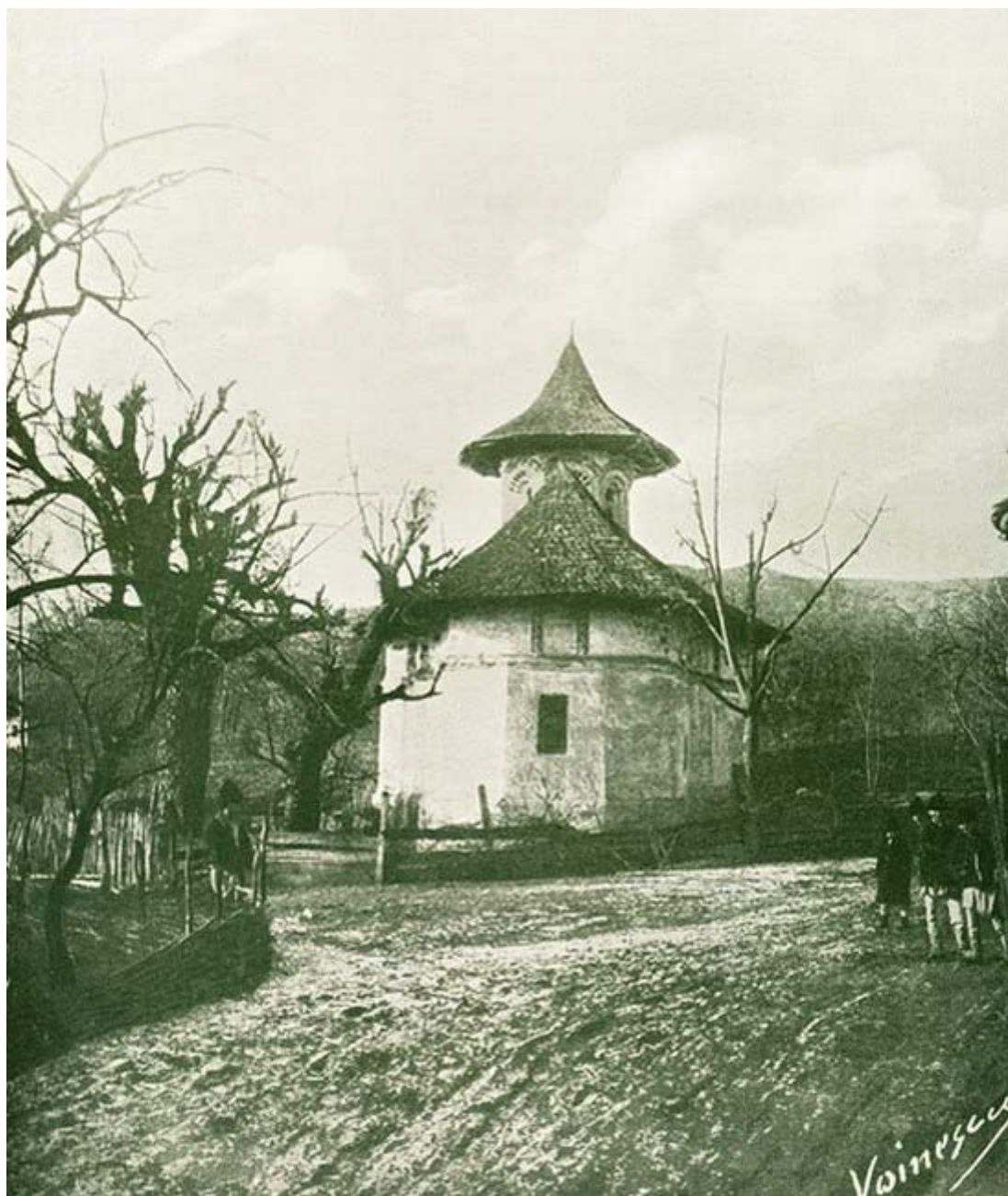
The roofs are always of shingle.
