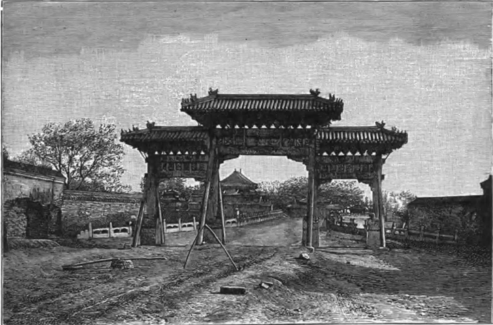
FIG. 944.—The Widows' Arch, Pai-lu , Gate of Honour, erected to the memory of a virtuous widow. Peking.
