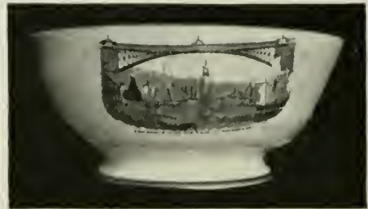
THE SUNDERLAND BRIDGE
