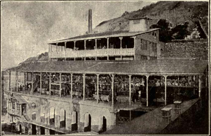
FIG. 69C.—SHOWING OPEN CONSTRUCTION OF MILL, MONTEPONI.
