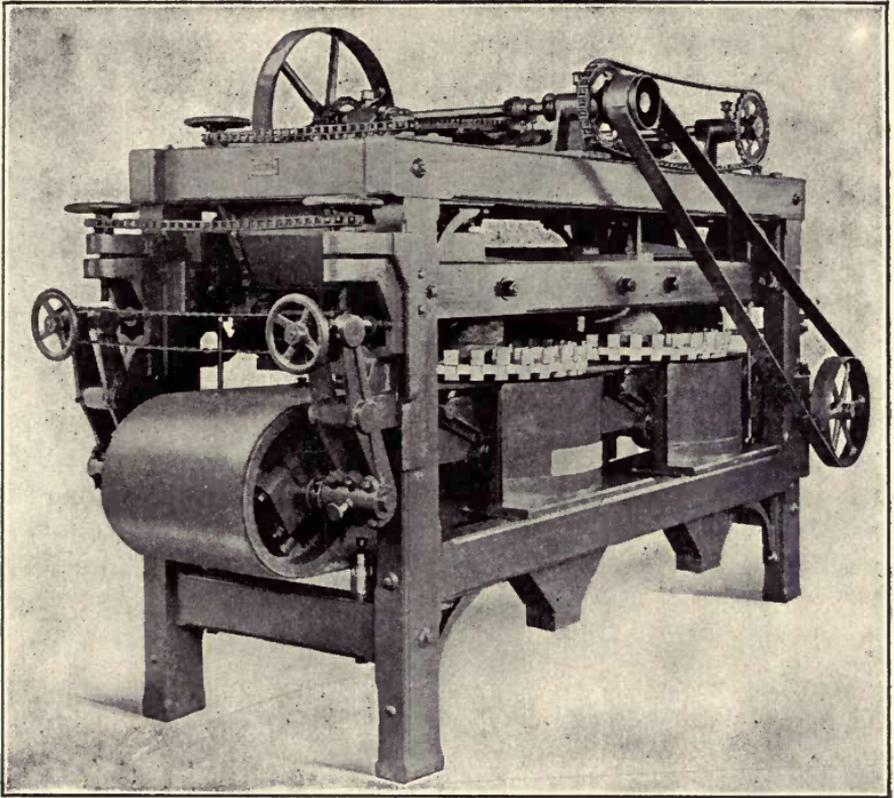
FIG. 19.—THE DINGS BELT TYPE SEPARATOR.
