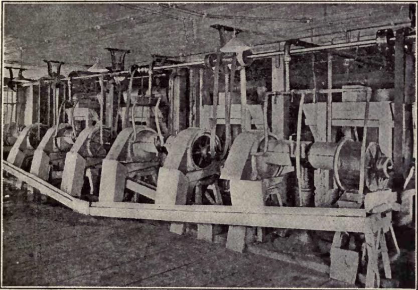
FIG. 55.—GRONDAL SEPARATORS AT HERRANG.
