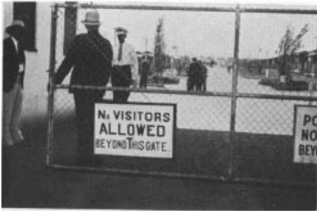
THE CONTROL GATE
