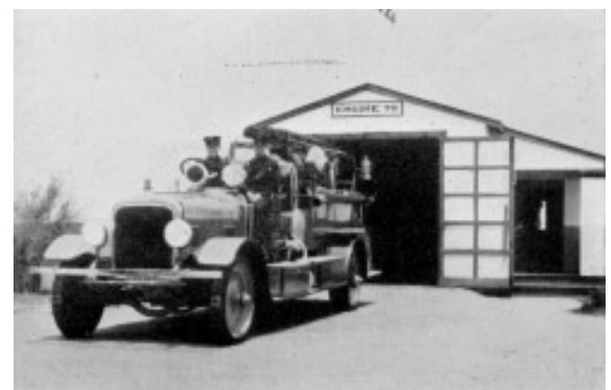
COMPLETE FIRE STATION
