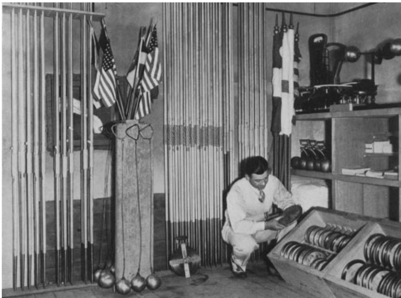
A CORNER IN THE EQUIPMENT ROOM, OLYMPIC STADIUM
