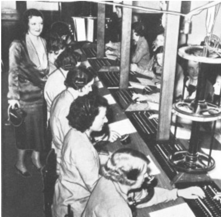
BATTERY OF TURRETS IN CENTRAL OLYMPIC TELEPHONE EXCHANGE
