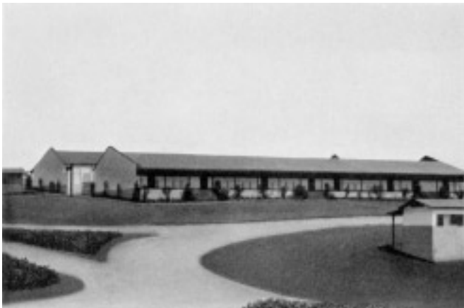
ONE OF COMPLETED DINING ROOMS
