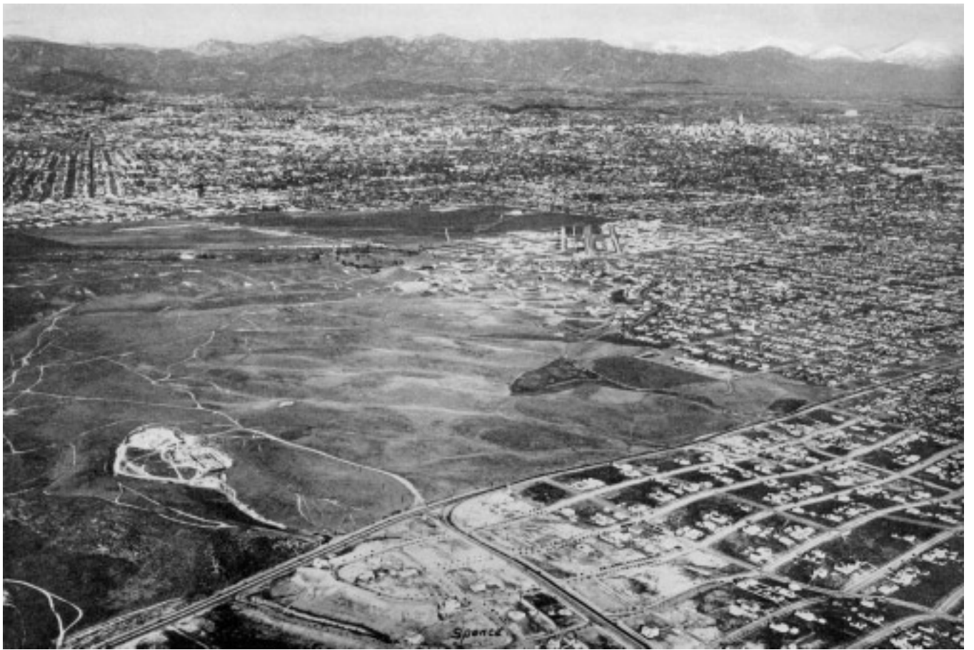
THIS AND FOLLOWING AIRPLANE VIEWS SHOW PROGRESS OF THE OLYMPIC VILLAGE CONSTRUCTION — ABOVE, THE BARREN HILLTOP
