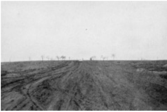
FIRST ROAD TO THE SITE
