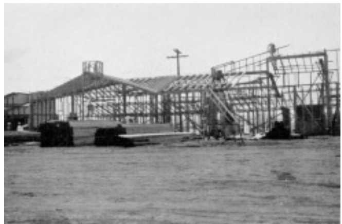
P'ORTION OF ADMINISTRATION BUILDING
