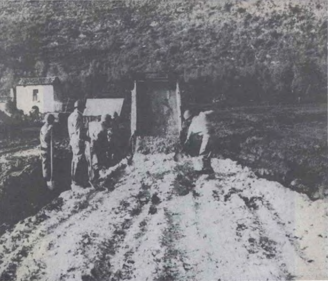
ENGINEERS SPREAD ROCK . . . .
