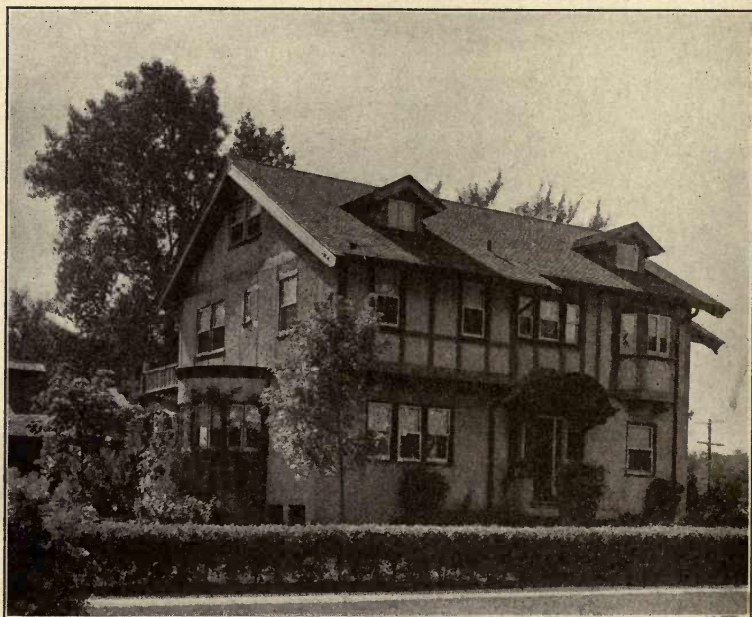
BUILT-IN GUTTERS LINED WITH COPPER.
