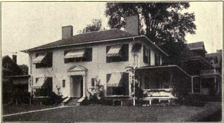
SHINGLE ROOF WITH HANGING METAL GUTTER.
