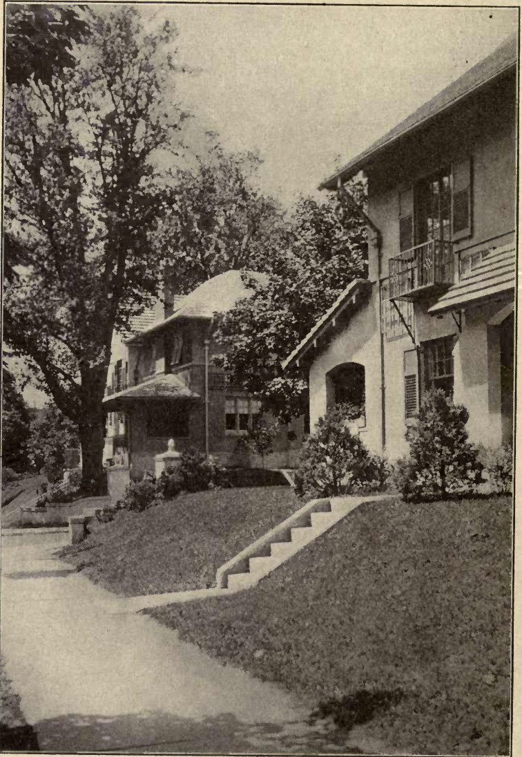
HOUSES IN A FIREPROOF COMMUNITY NEAR NEW YORK. Mann and MacNeille, Architects.
