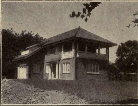
LARGE BRICK GARAGE.
