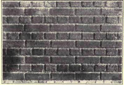
BRICKWORK LAID IN ENGLISH BOND.
