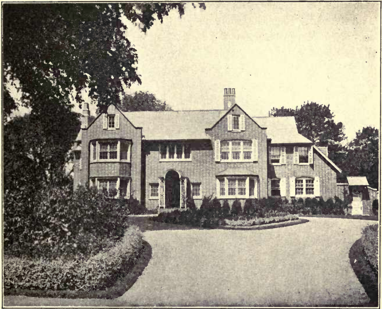
BRICK COUNTRY HOUSE NEAR BOSTON.
