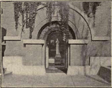
MOLDED BRICK ARCH OVER AN ENTRANCE.
