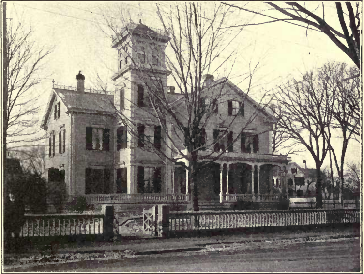
OLD HOUSE BEFORE REMODELING.
