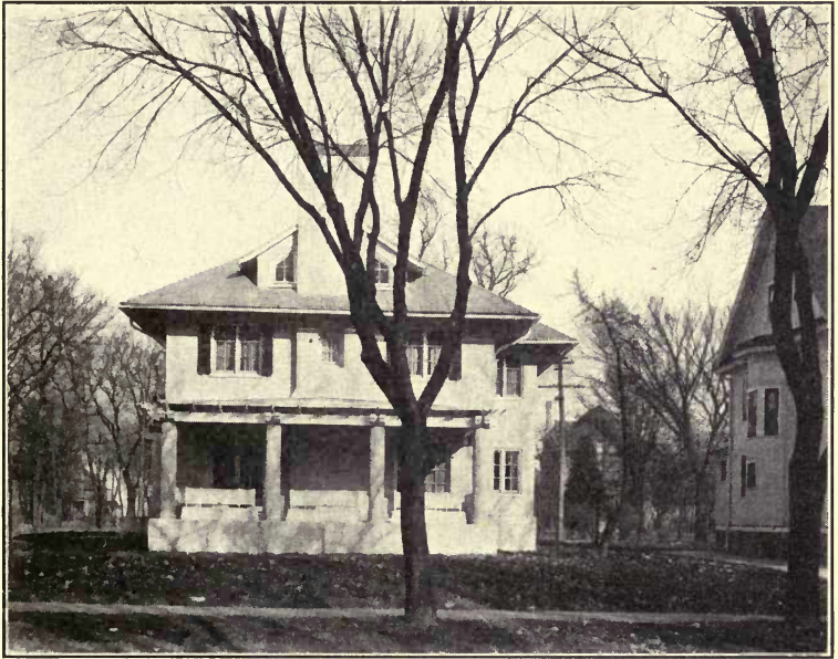
VERANDA ON END OF HOUSE.
