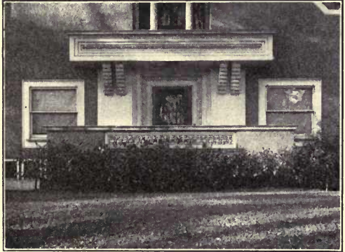
DOME LIGHT AT ENTRANCE.
