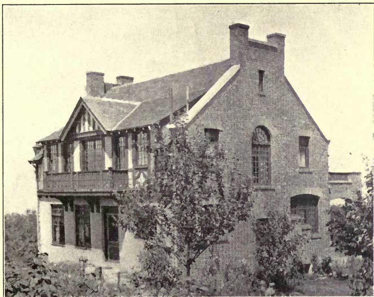
PLUMBING STACKS EXTENDING ABOVE ROOF.
