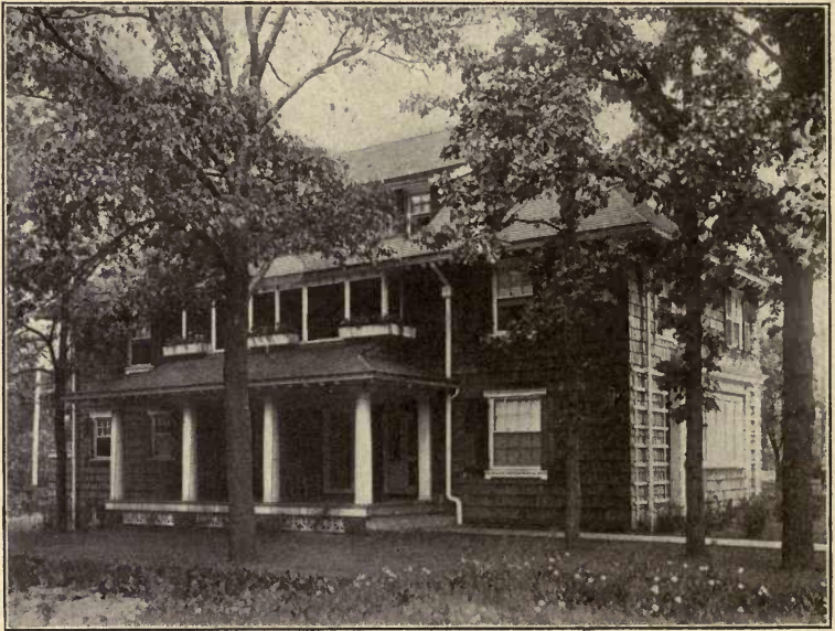
GALVANIZED IRON GUTTER AND CORNICE.
