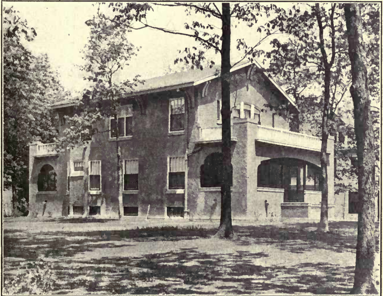
STEEL FRAME HOUSE COMPLETED.
