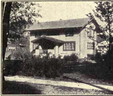
CEMENT-PLASTERED HOUSE OF MODERATE COST.
