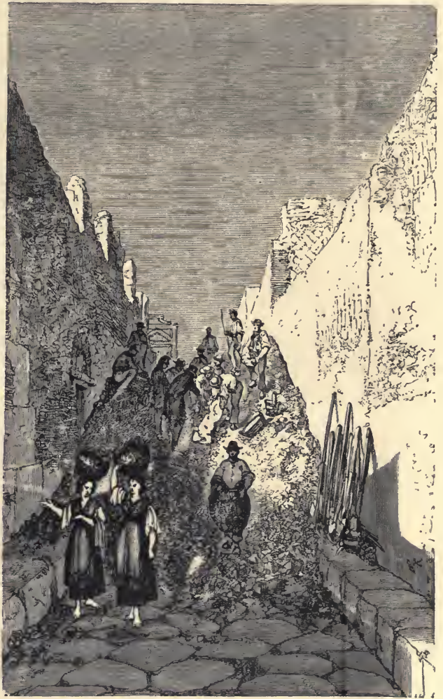
CLEARING A STREET.
