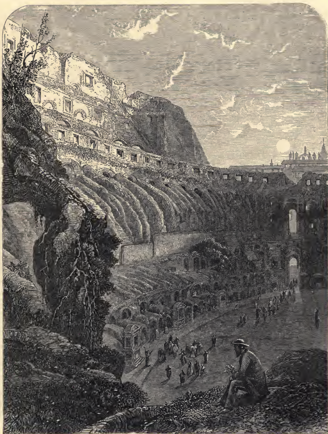
THE COLOSSEUM BEFORE THE RECENT EXCAVATIONS.
