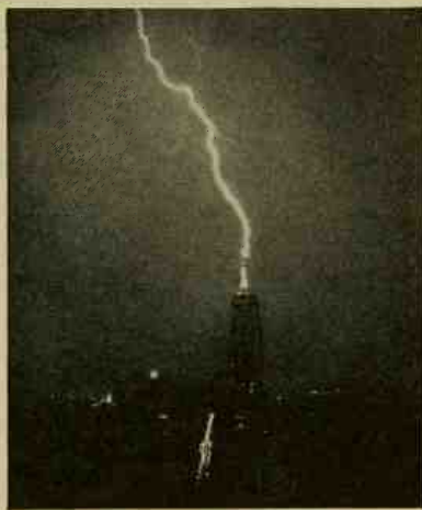
FIG. 233. Lightning striking the Empire State Building, New York City. Although this building has been struck by lightning many times, no harm was done to the building because its steel framework acts as a Faraday cage. (Courtesy of the General Electric Company.)
