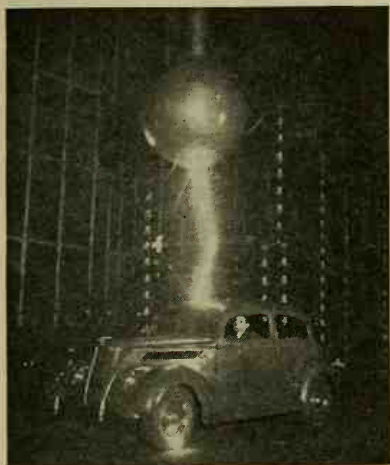
FIG. 232. Three million volts of laboratory lightning striking a car in the Westinghouse high voltage laboratory. The bolt can be seen jumping over the left front wheel to reach the ground. (Courtesy of the Westinghouse Electric and Manufacturing Company.)
