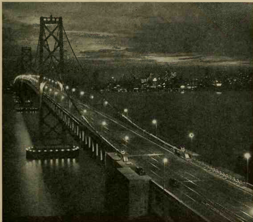
FIG. 174. Sodium vapor lamps illuminate the San Francisco-Oakland Bay Bridge. (Courtesy of the Pacific Gas and Electric Company.)
