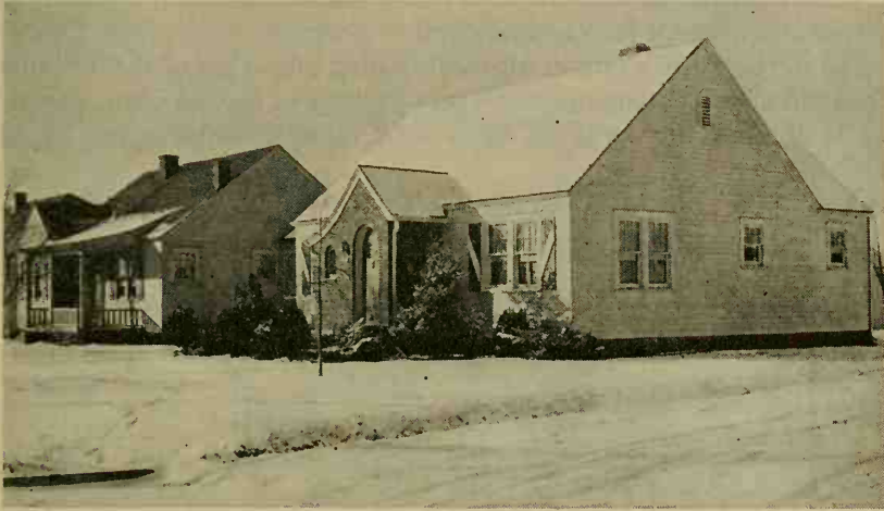
FIG. 90. The house on the right has been insulated while the house to its left has not been insulated.
