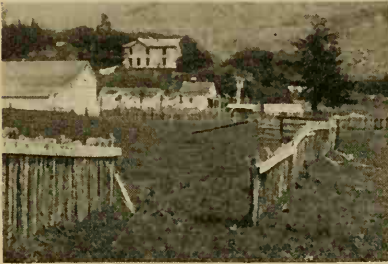
FIG. 43. A fence shifted by an earthquake. (Courtesy of the U. S. Geol. Survey.)
