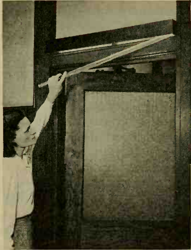
FIG. 176. This yard-long germicidal lamp promptly destroys a high percentage of the bacteria borne by air currents through this doorway. (Courtesy of the General Electric Company.)
